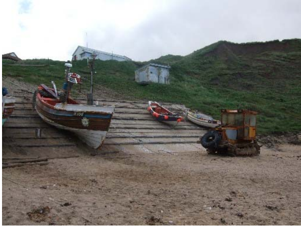
Concrete revetment (Asset Ref No. 1221D901D1803C02)
