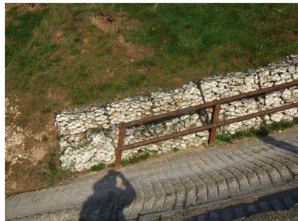
Gabions along edge of Lifeboat slipway (Asset Ref No. 1231D901D3201C03)
